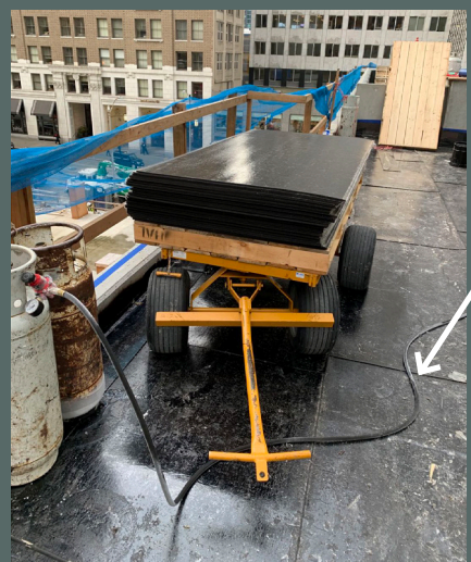
Gas hose (Other conduits, electrical cords, or pipelines can also become obstacles.)
