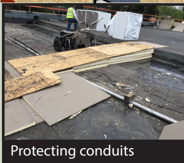
Bridging gaps between two levels of roof
