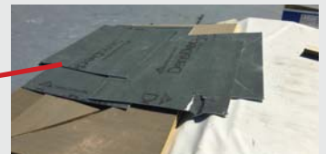
Uneven running slope built with DensDeck and ISO
