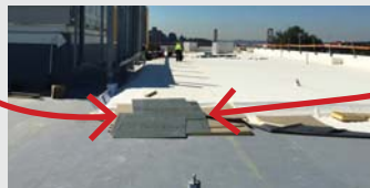
Loose or unsecured ramp materials create gaps
